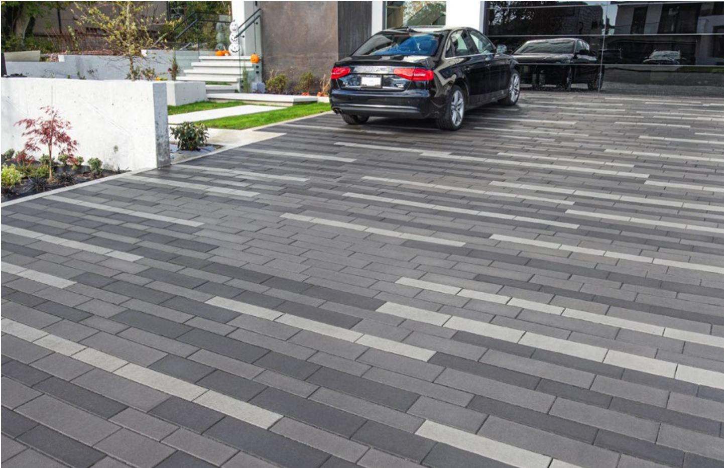
Photo courtesy of Ratan Raymon Construction Ltd. Silver Grey, Midnight Black, and Graphite laid together. Pattern achieved by ordering pallets of three different colours.
