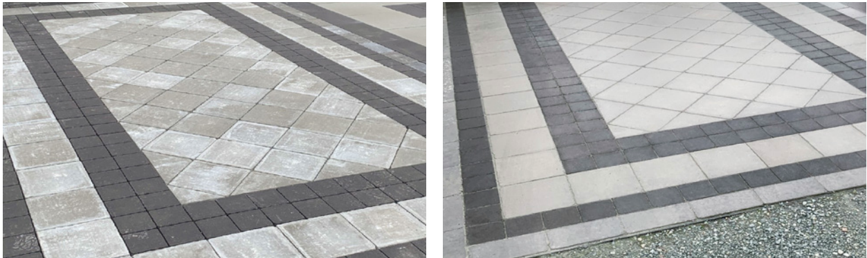
Two images displayed above depict the project's progression over a 9-month timeline, showcasing the initial state and the final outcome achieved without any cleaning intervention.
