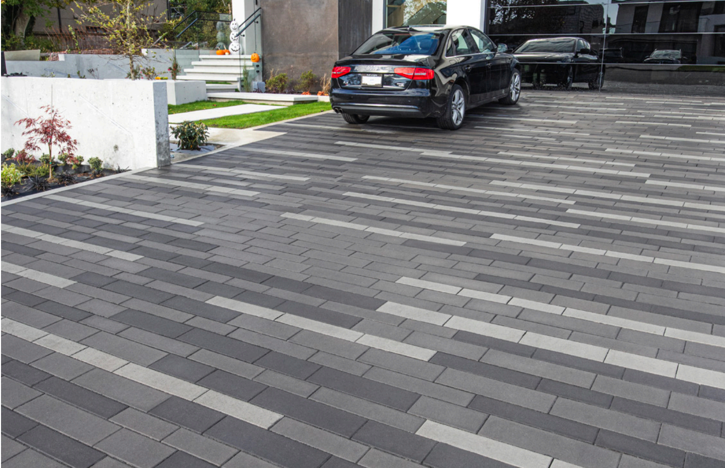
Photo courtesy of Ratan Raymon Construction Ltd.
